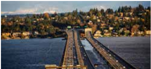
2. I-90 FLOATING BRIDGE.
