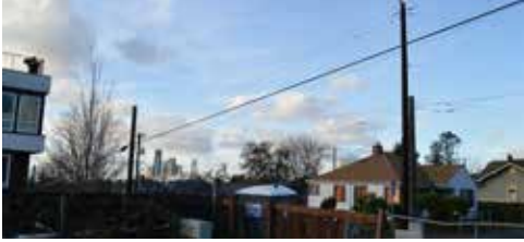
5. VIEW TO NORTH WEST.
