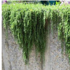
Spiller landscaping at retaining wall planters (DC4.4.A Plant Materials & Hardscape)
