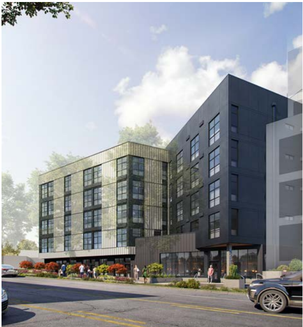
5231 Rainier Ave S (Under Construction)
