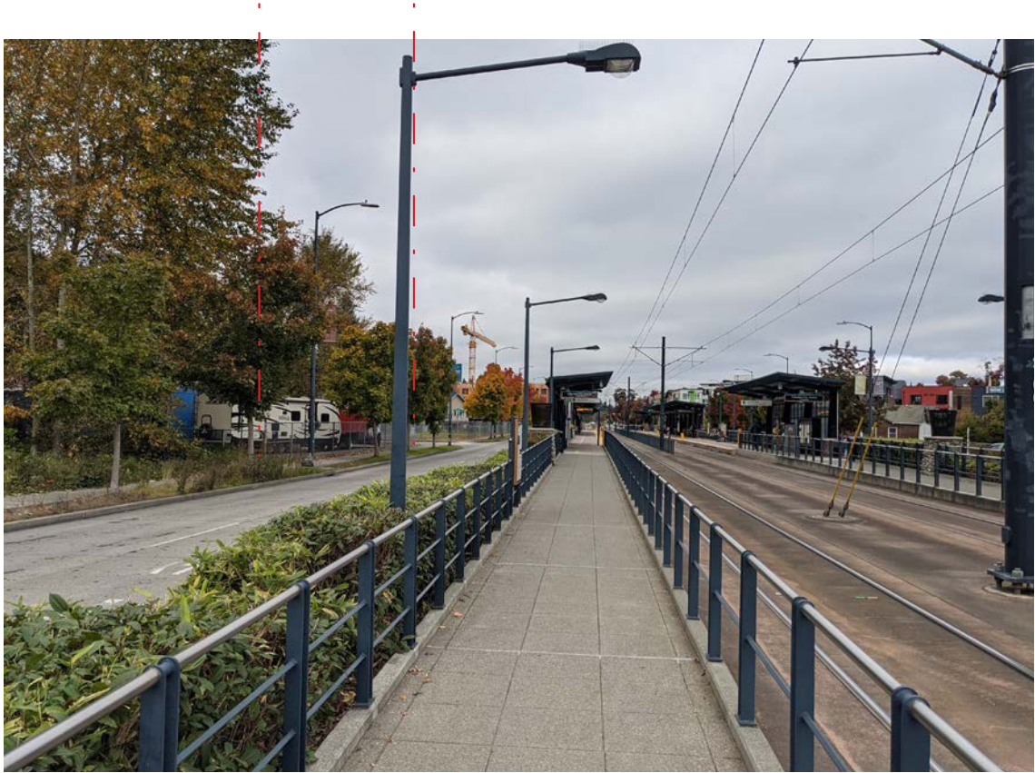
1. Looking north on light rail platform
