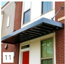
11 Metal Channel Canopy, Black Powdercoat
