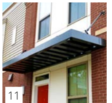
11 Metal Channel Canopy, Black Powdercoat
