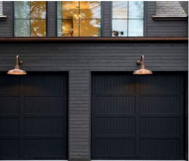
GARAGE DOORS + LIGHTING
