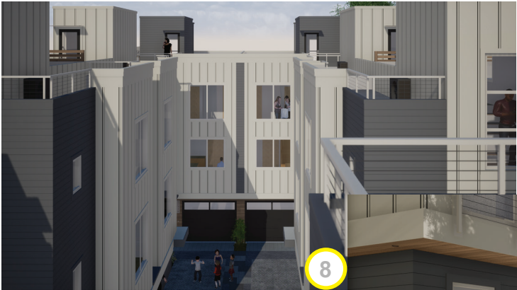
UNIT 2 DECK - FACING WEST
