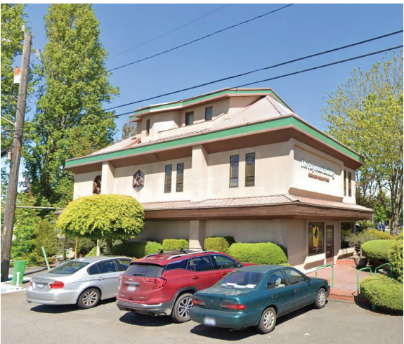
HAYWOOD BLDG. (ON 14TH)
