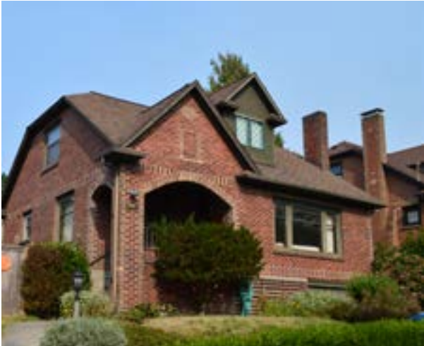
NEARBY VINTAGE BRICK HOUSE
