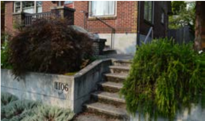
STAIRS AT UPHILL YARDS - STAIRS TURN AT LANDING - USE OF BRICK AND CONCRETE
