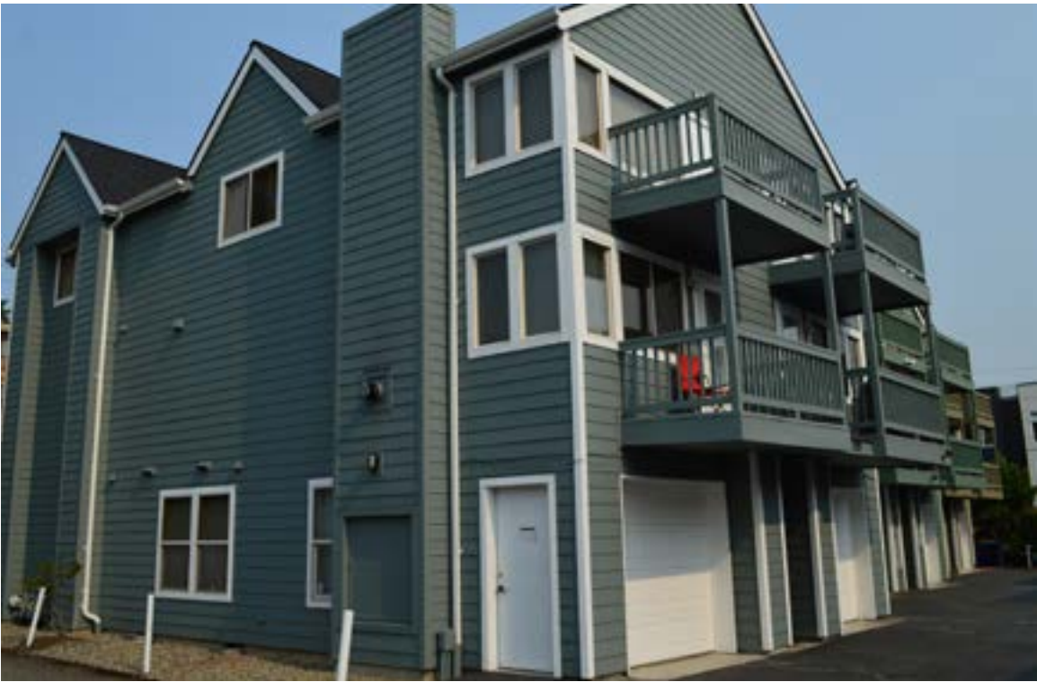
HOMES ADJACENT TO ALLEY
