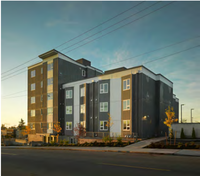
EvCC Student Housing Everett, WA 120 Units
