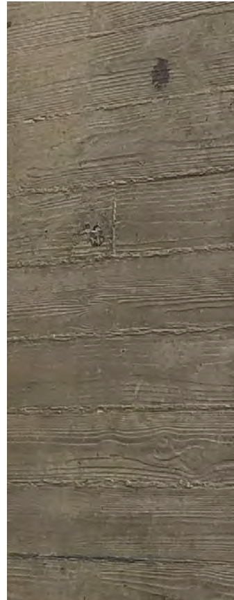
Example of Concrete w/ Graffiti Coating
