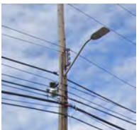
SL-1 Existing Pole mounted "Cobra head" Street Light
