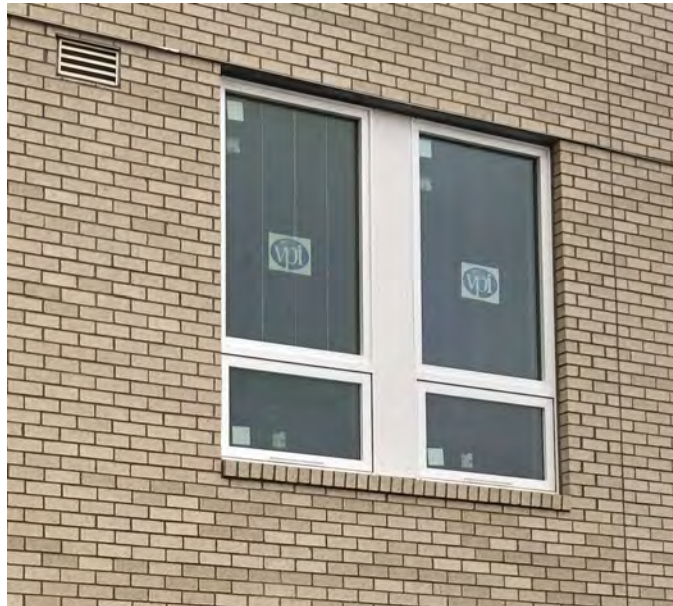
Example of vinyl flanged window with proposed brick detailing.
