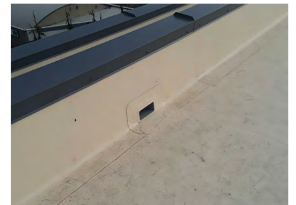
Tan TPO Roofing
