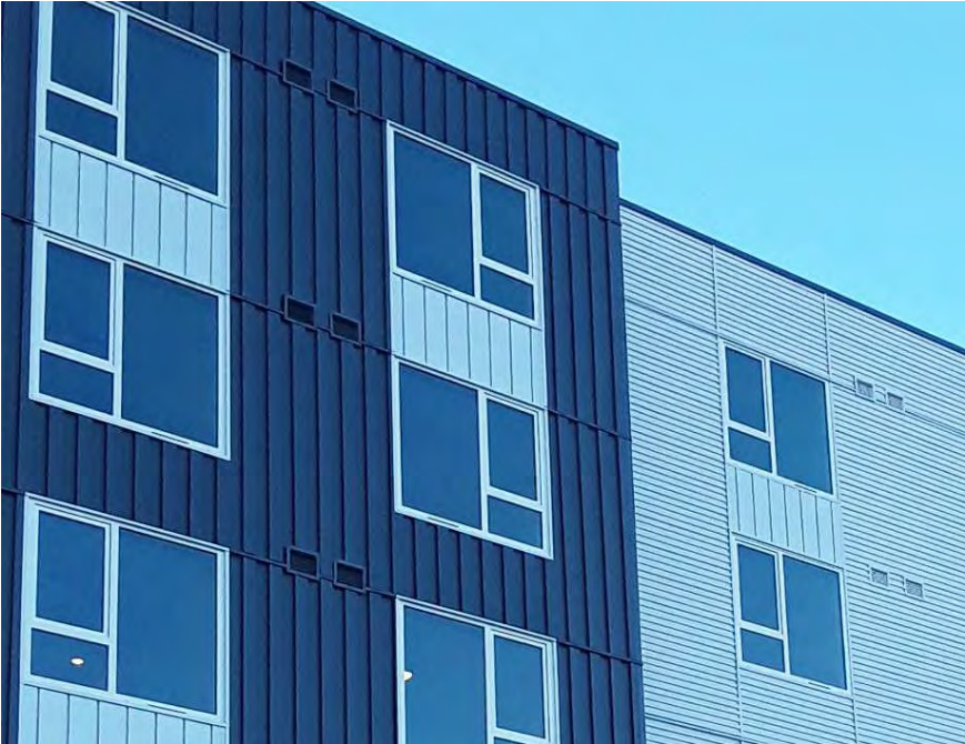
Color Matched Xvent Installation in Metal Siding
