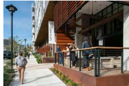
Example of an eroded corner with street level patio.
