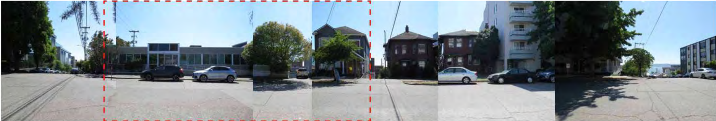
B: West Republican Street Elevation Looking south.
