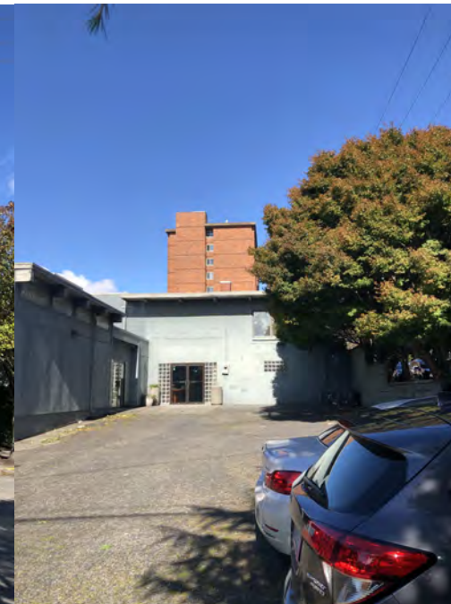
J) Existing wood and masonry building.
