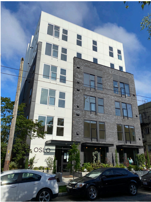
PHOTO OF COMPLETED EAST ELEVATION SHOWING SIMPLIFIED MATERIALS. NOTE: INCREASED ROOFTOP ELEMENTS ARE NOT VISIBLE FROM THE STREET LEVEL.
