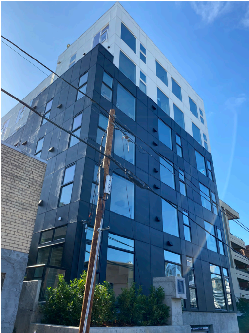
PHOTO FROM ALLEY SHOWING CONTINUOUS 4-STORY BASE AND SIMPLIFIED FACADE (SOUTHEAST CORNER)
