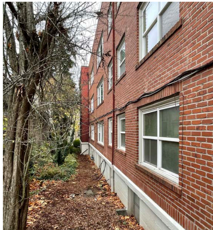
VIEW FROM WEST (13TH & 14TH ST ALLEY)
