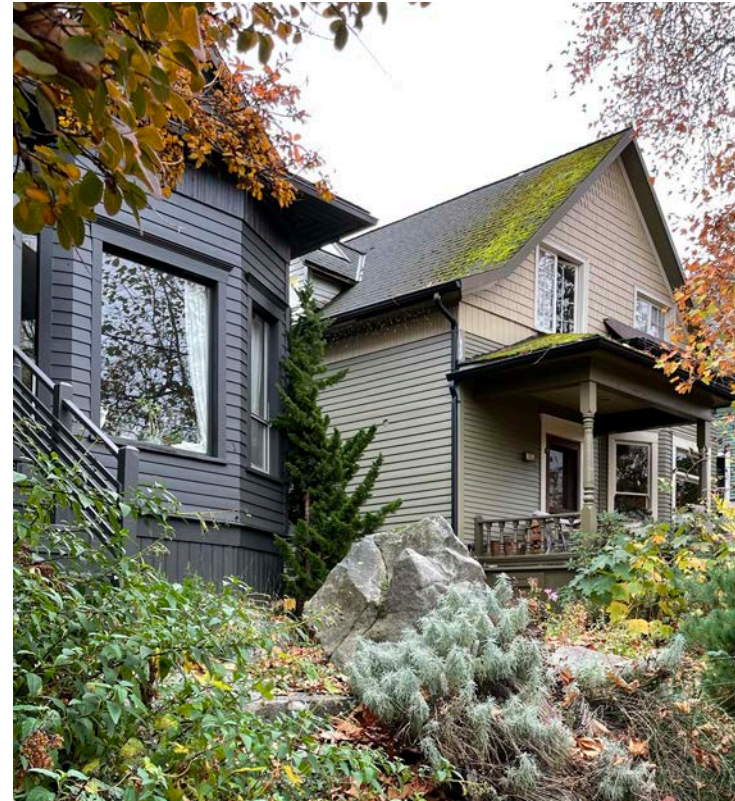
VIEW FROM NORTH (13TH ST)
