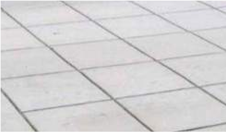
1: SDOT Standard Concrete 2'X2' scoring and sawcut joint
