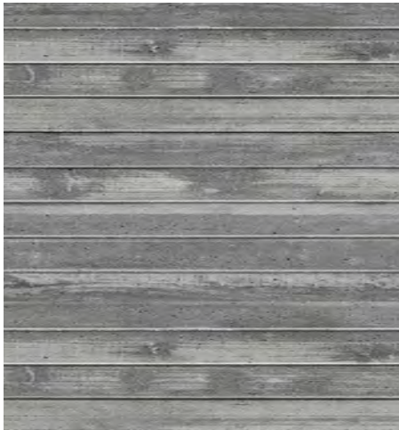
CON-1 Board-form concrete, 8" seams
