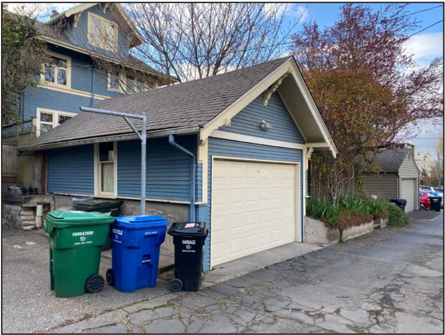
EXISTING SITE STRUCTURES LOOKING NW
