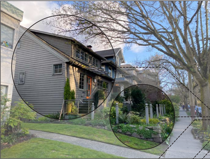
EXISTING SITE STRUCTURES LOOKING SE
