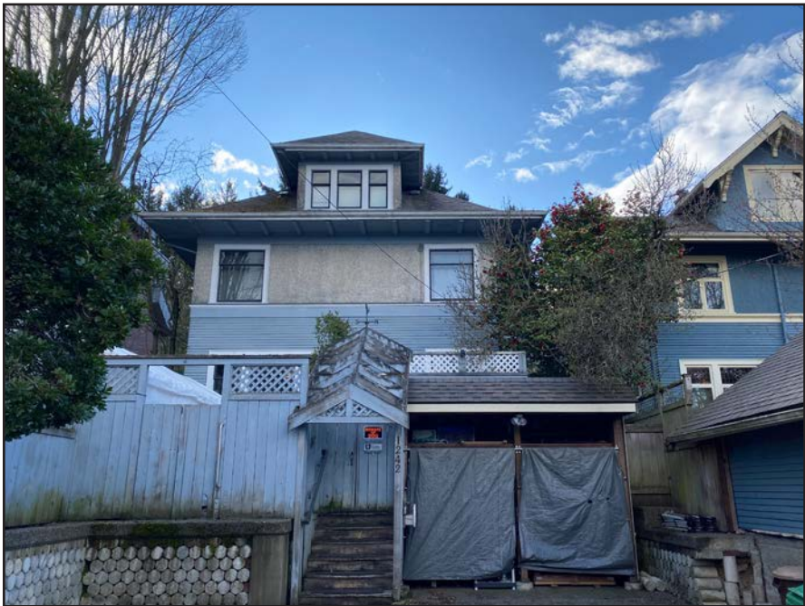
EXISTING SITE STRUCTURES LOOKING W
