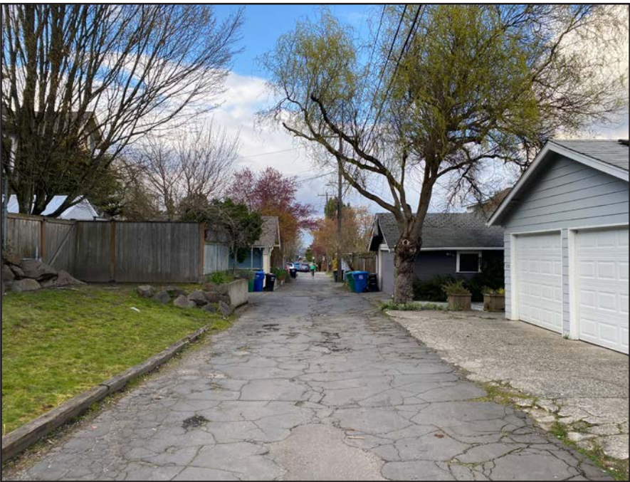
EXISTING ALLEY LOOKING N
