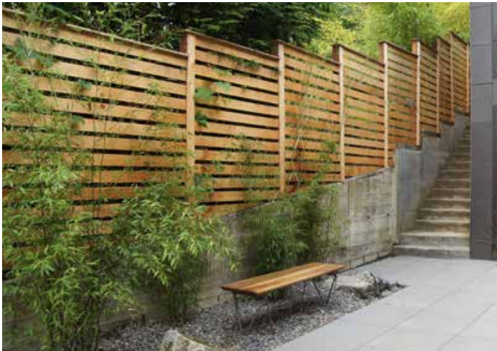
(B) Landscaped spaces into the alley
