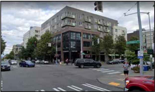
All way pedestrian crossings at transit hub
