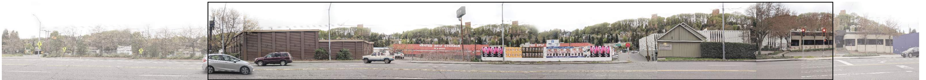
ACROSS FROM SITE
