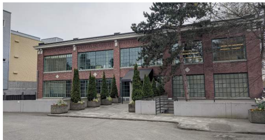
⑧ LOOKING SE FROM PARKING LOT TOWARDS BLACK MANUFACTURING BUILDING
