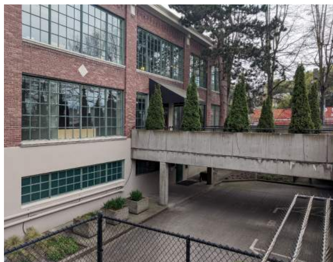
⑦ LOOKING SE FROM PARKING LOT TOWARDS BLACK MANUFACTURING BUILDING
