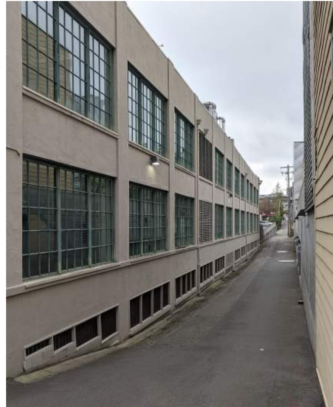
ALLEY EAST OF BLACK MANUFACTURING BUILDING
