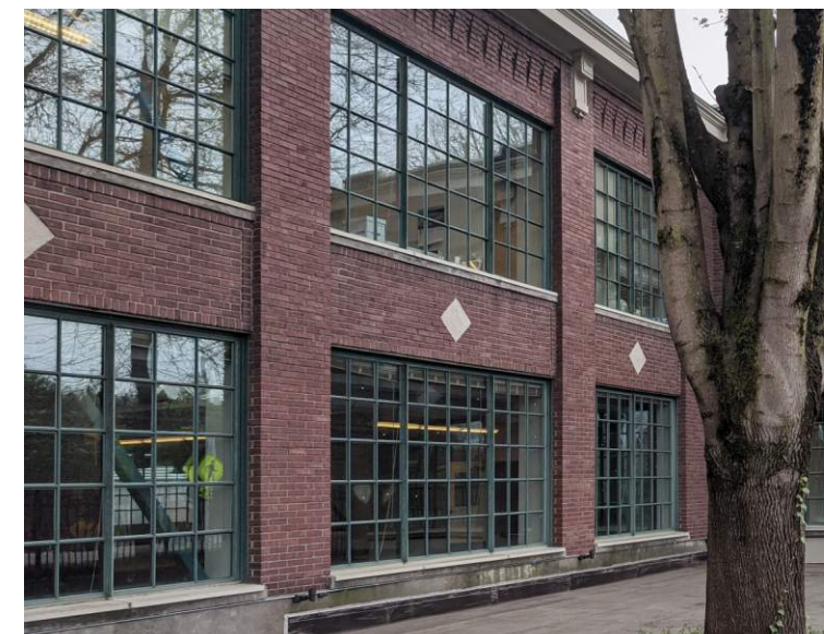
STRUCTURAL (PIER) ELEMENTS ARE BROUGHT TO THE FRONT
