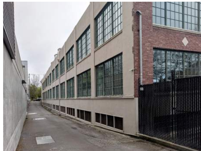
⑤ LOOKING SOUTH ADJACENT TO SITE IN ALLEY
