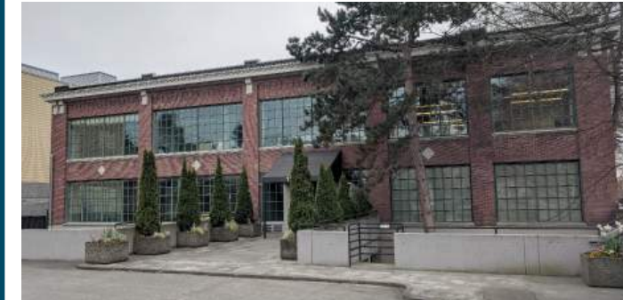
PRESERVING EXISTING STRUCTURES
