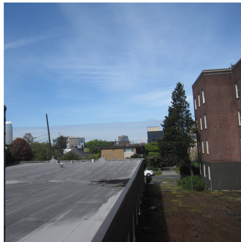
5 / BETWEEN EXISTING AND PROPOSED BUILDING LOOKING WEST
