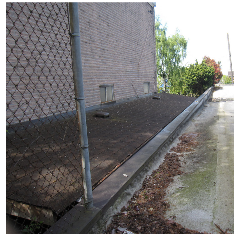
6 / SOUTH PROPERTY LINE LOOKING WEST
