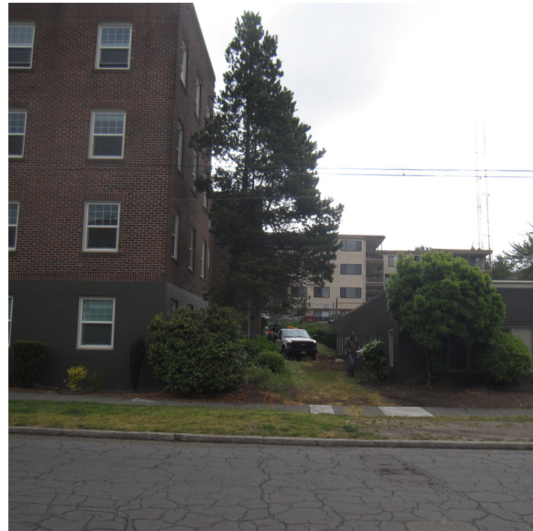
2 / BETWEEN EXISTING AND PROPOSED BUILDING LOOKING EAST
