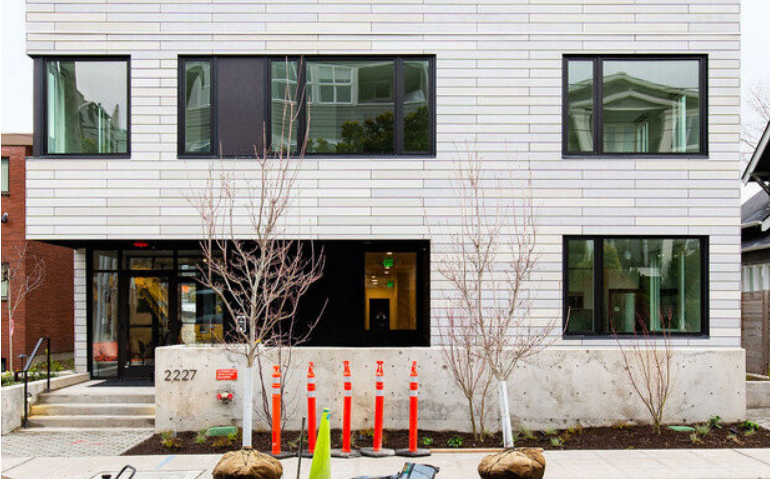
SMALL SCALE MATERIAL WITH PUNCHED OPENINGS
