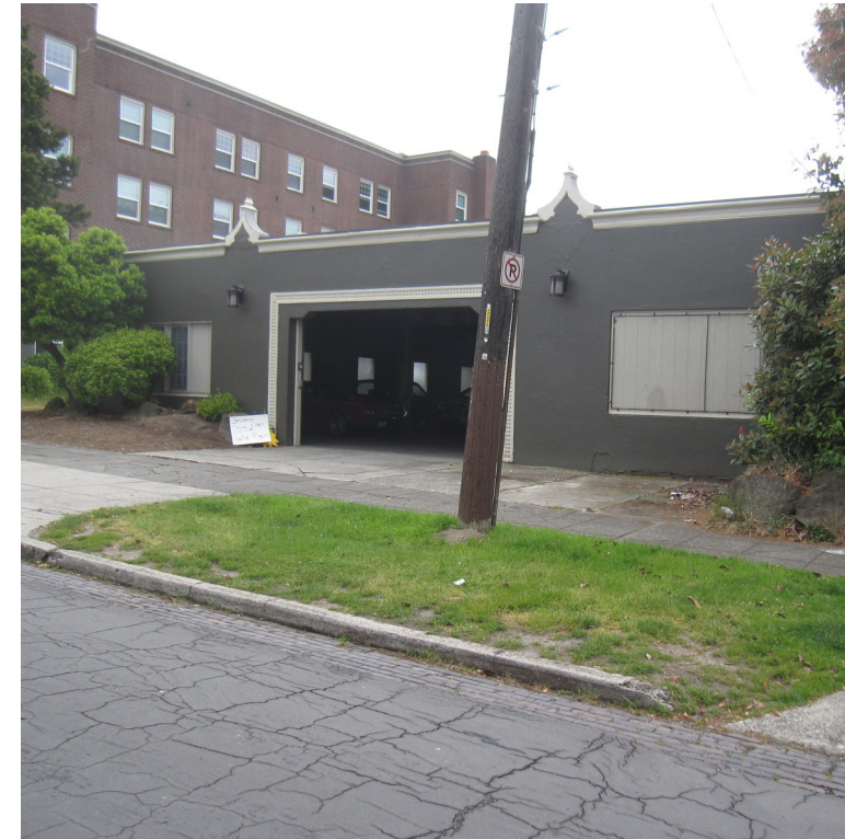
3 / LOOKING NE FROM 13TH AVENUE
