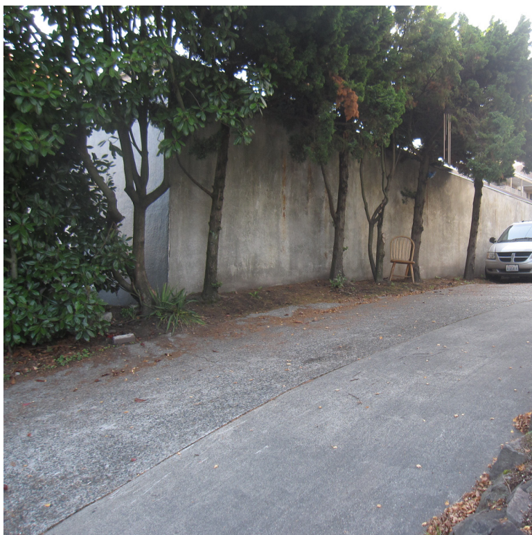
4 / SOUTH PROPERTY LINE LOOKING EAST
