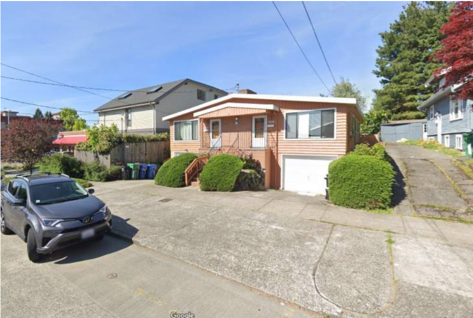
LOOKING SOUTHWEST ON SUNNYSIDE AVE N, ADJACENT NEIGHBOR TO SOUTH SHOWN
