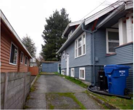
EXISTING DRIVE FACING WEST
