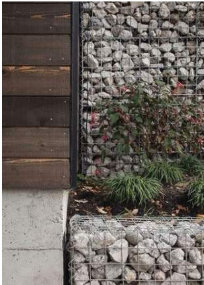
Integration of Gabion walls, concrete, cedar siding
