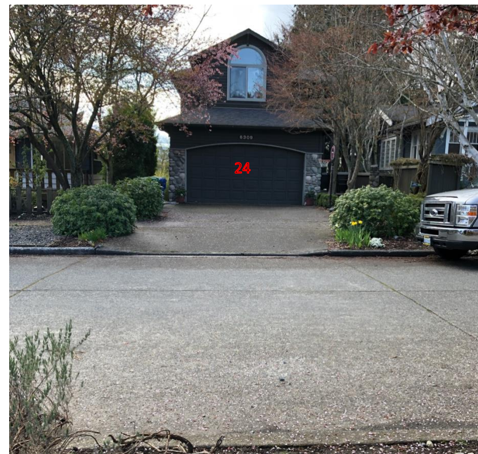
Zoned LR3 (located on west side of 41 st Ave SW, south of Graham St.)
