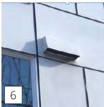
6 Venting Shroud, Painted to Match Field
