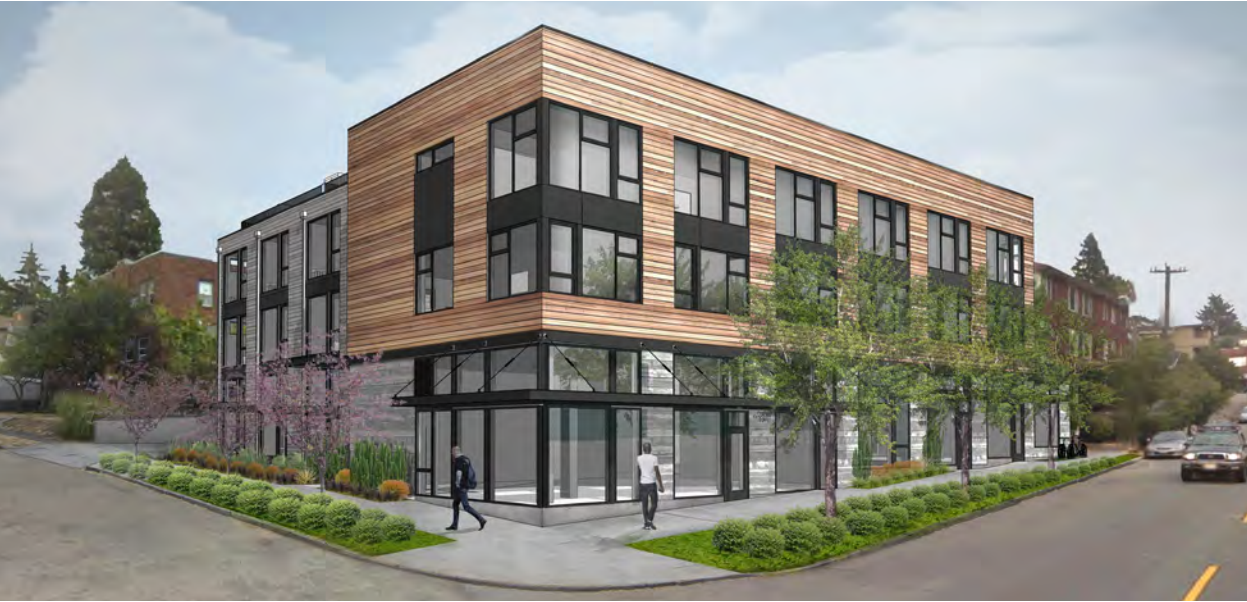
412 NW 65th St (Under Construction)
