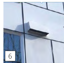
6 Venting Shroud, Painted to Match Field
