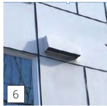
6 Venting Shroud, Painted to Match Field
