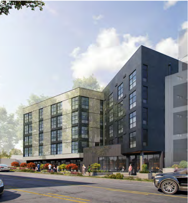
5231 Rainier Ave S (Under Construction)
