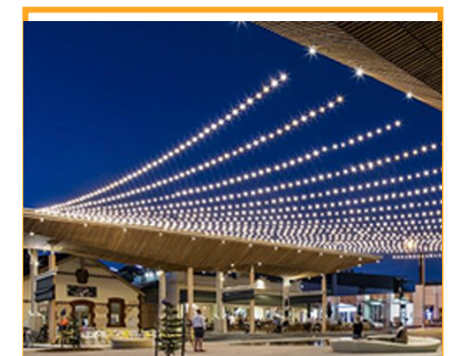
J CATENARY LIGHTING
