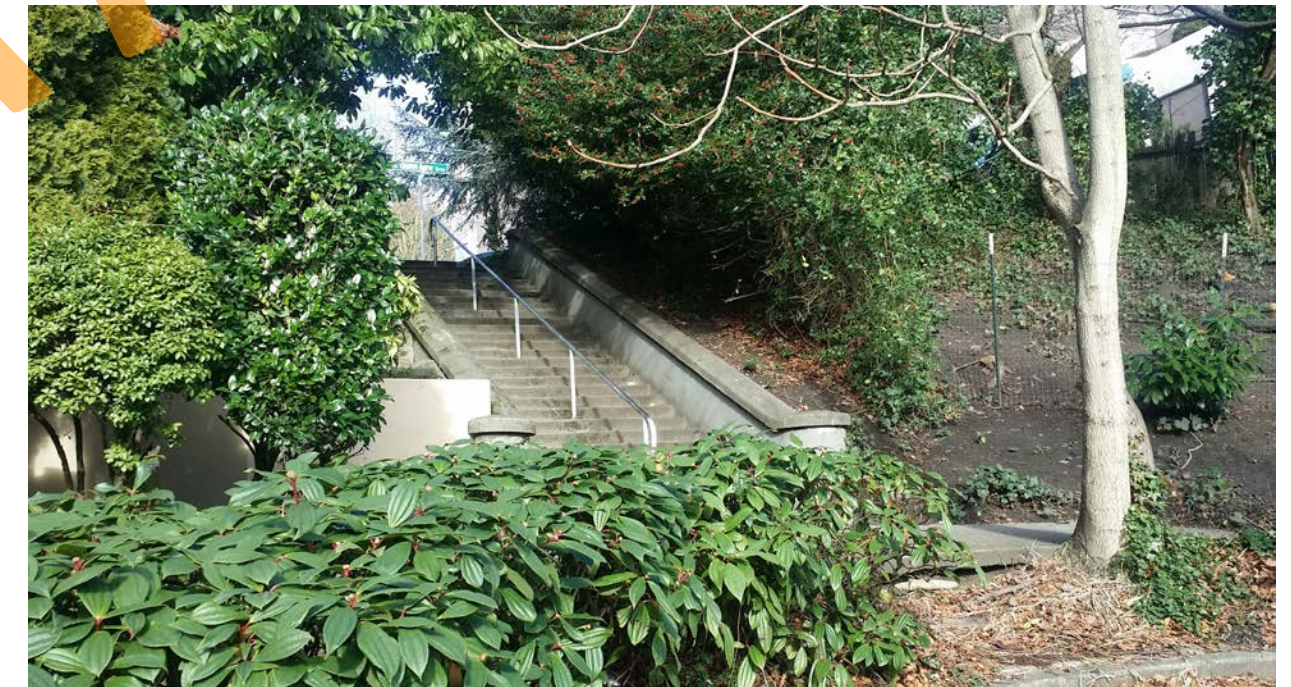
D PEDESTRIAN STAIRCASE CONNECTING 1ST AVE W AND W. QUEEN ANNE DRIVEWAY
