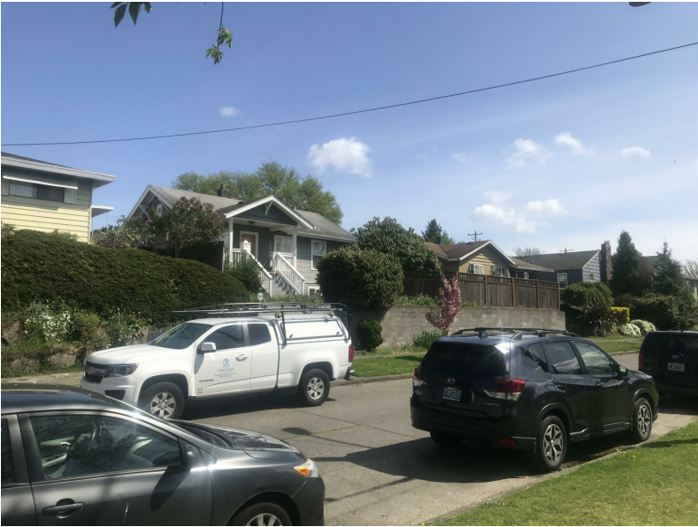
VIEW OF SITE FROM NW
