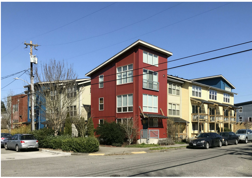
2 - NE CORNER OF 18TH AVE SW AND SW BARTON ST THREE STORY MULTIFAMILY
