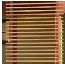
CLEAR STAINED CEDAR SCREEN WALLS
