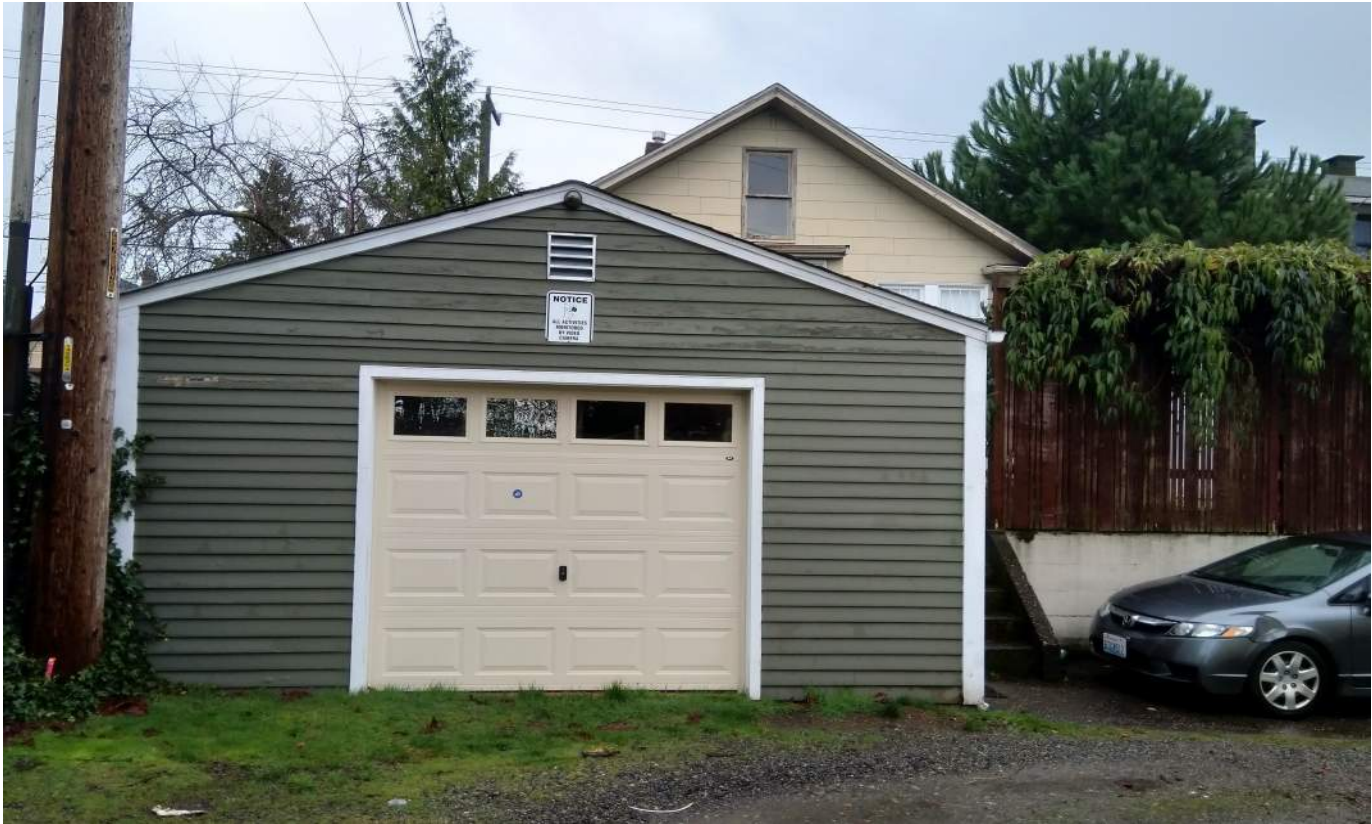
EXISTING WEST ELEVATION FROM ALLEY
