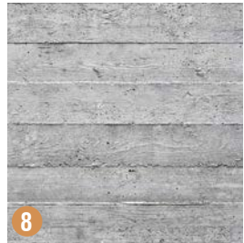
board formed concrete
