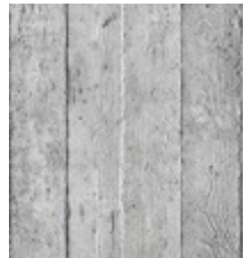
1 BOARD FORM CONCRETE
