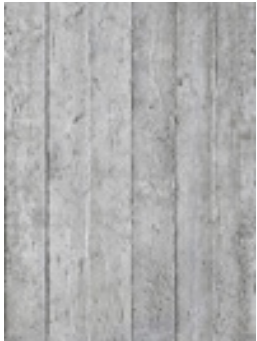
6 BOARD FORM CONCRETE
