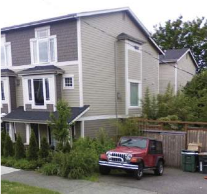
2 ADJACENT BUILDING - SOUTH
