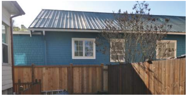
4 ADJACENT BUILDING - SOUTH
