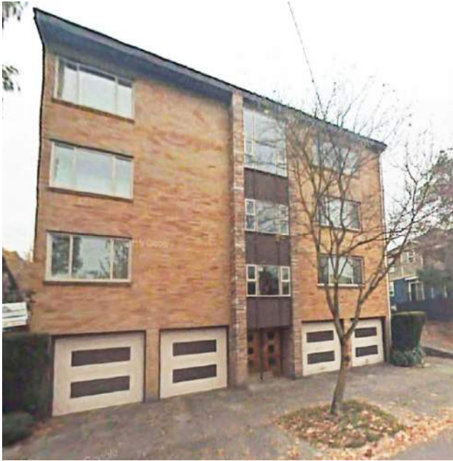
3 ADJACENT BUILDING - EAST
