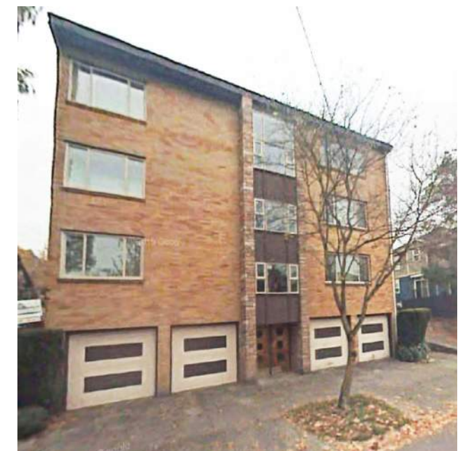
3 ADJACENT BUILDING - EAST
