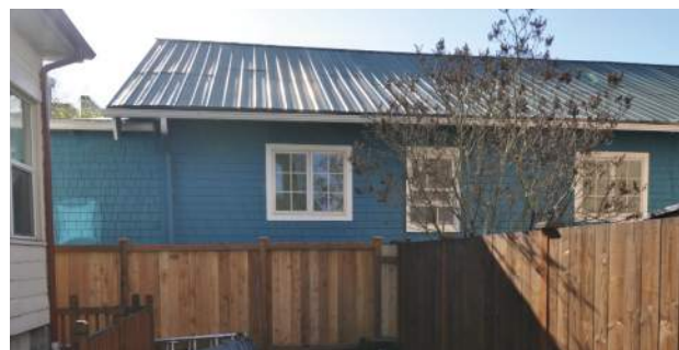
4 ADJACENT BUILDING - SOUTH
