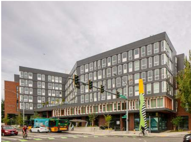
Neighbor Apartment Building - Mixture of Bricks and Cement Board
