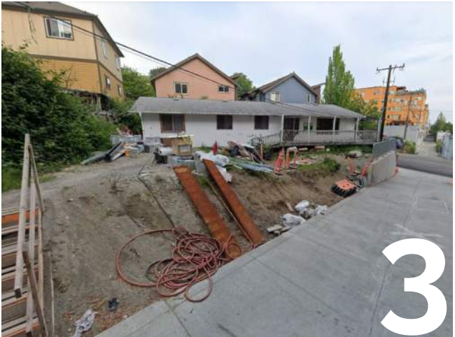
W View of the Site (from Alley)
