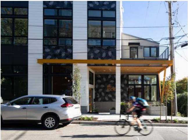
The Roost Apartments - Setback Entrance with Cantilever
