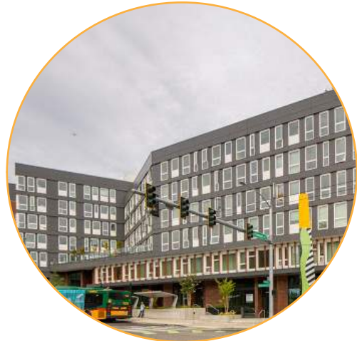
Muir Apartment - A mixed-use apartment at the corner of Rainier Ave S and S Dearborn St. shows variety of material choices including bricks, cement board, and corten metal.
