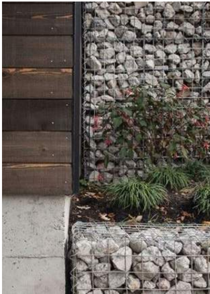
Integration of Gabion walls, concrete, cedar siding
