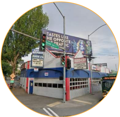
Automobile Shop - Commercial building right across the street from the site. Rough material.
