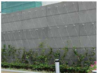
CABLE TRELLIS VEGETATED WALL
