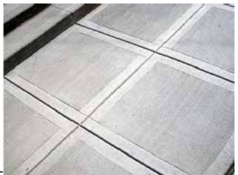
2X2 CONCRETE SCORING
