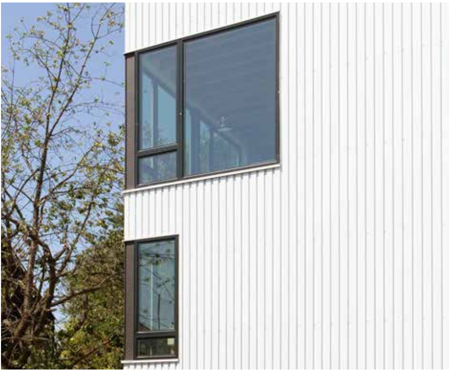
Box Rib Metal Siding Metal Sales T16-L Wall - "Snowdrift"
