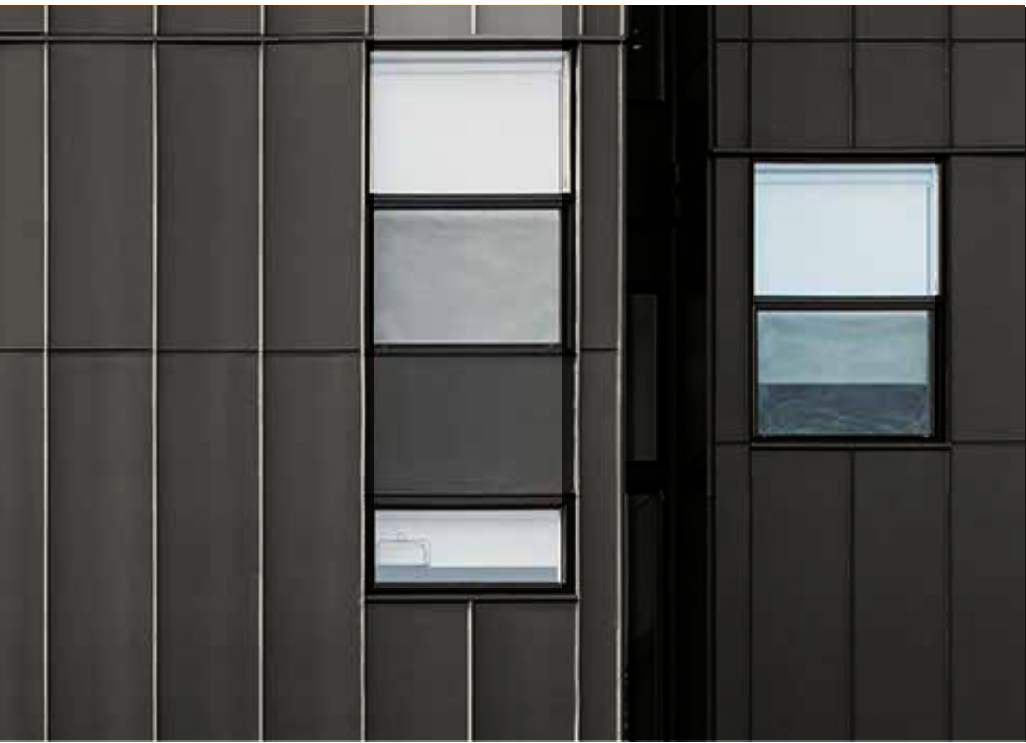
Fiber Cement "Standing Seam" with projected flashing profile in "Seal Skin" SW 7675
