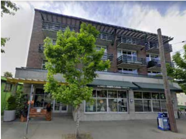
LARGE ROOF OVERHANG WITH DEEP RECESSED ENTRY
