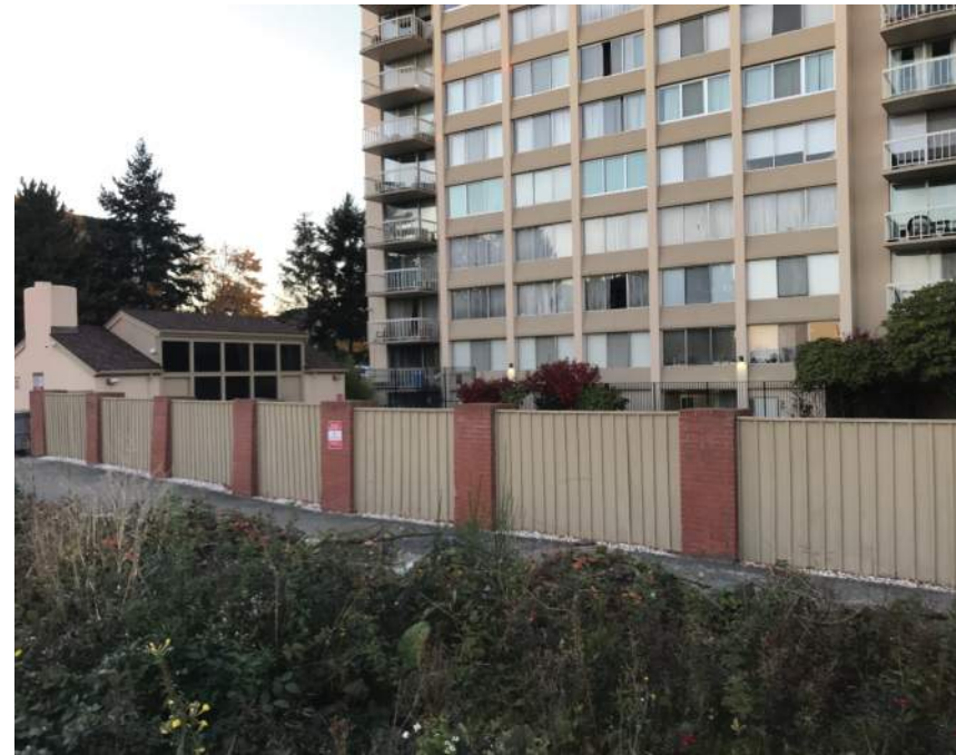
EXISTING CONDITION AT NORTH ALLEY
