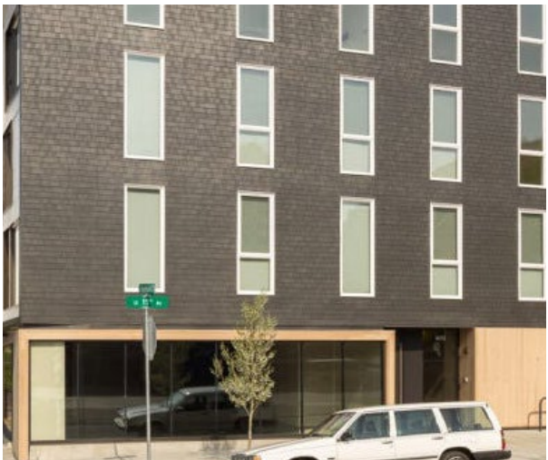
Simple and elegant upper facade with repetitive window pattern. Contrasting lower facade for commercial use.
