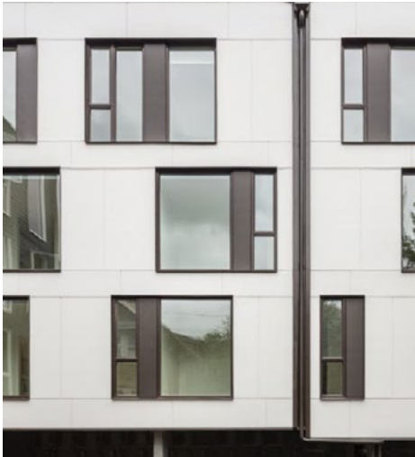
An elegant modern facade design with a simple building massing with playful window patterns
