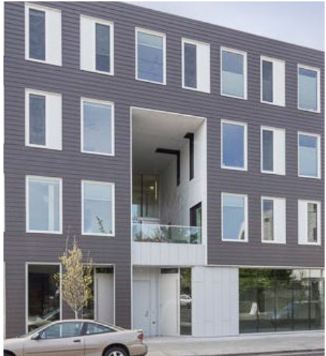
A facade pattern with a difference size of fenestrations and minimal use of colors. Outdoor common amenity open to street.
