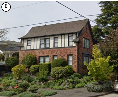
Existing low-rise residential structure. The unique use of brick pattern and hierarchy in facade design.
