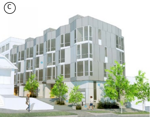
Planned 4 story multi-family structure. Street level facade along Aurora Ave N is decorative screen for parking without commercial use. Upper level fenestration pattern is unique.
