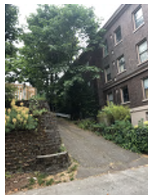
Partial View of South Building Facade
