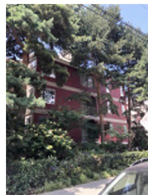
Partial View of North Building Facade
