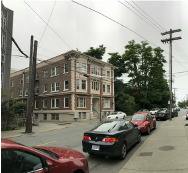
South Adjacent Structure
