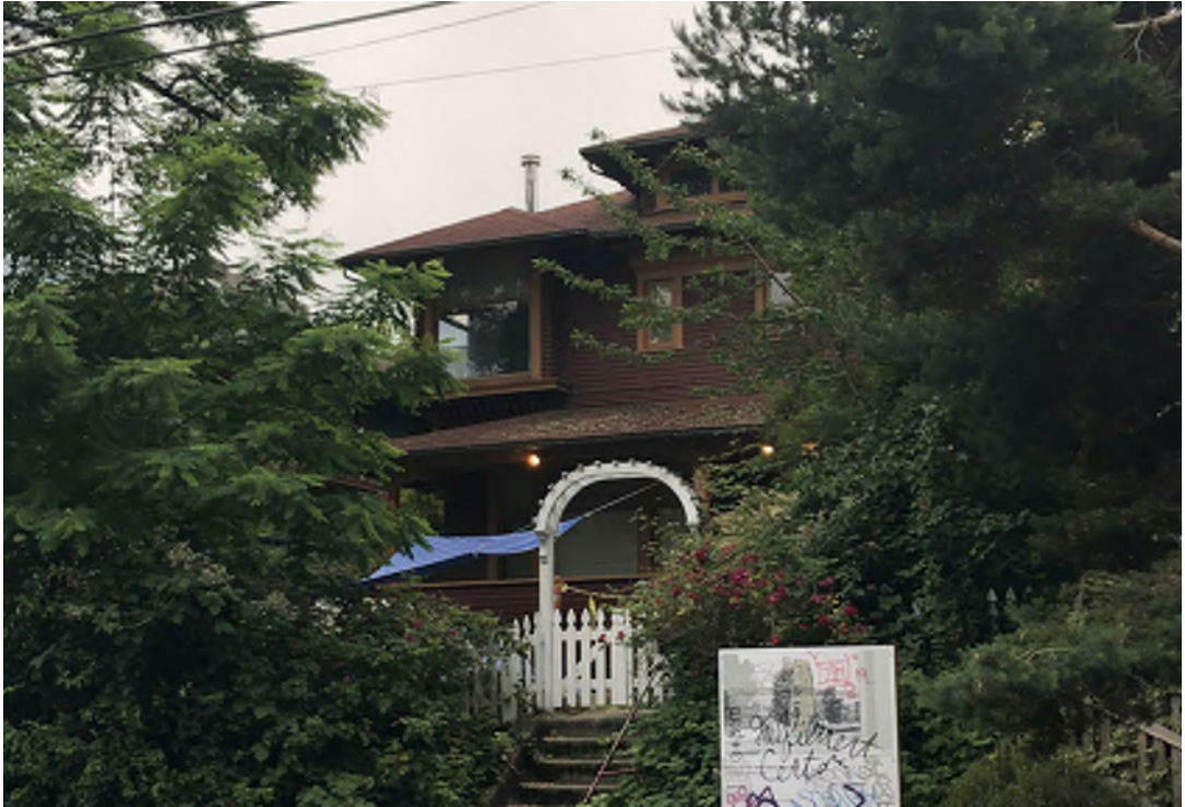
Exist. Structure A
