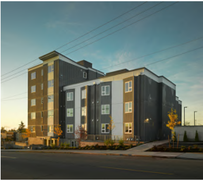
EvCC Student Housing Everett, WA 120 Units
