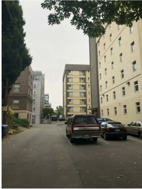
West Structure in Alley Adjacent to Site
