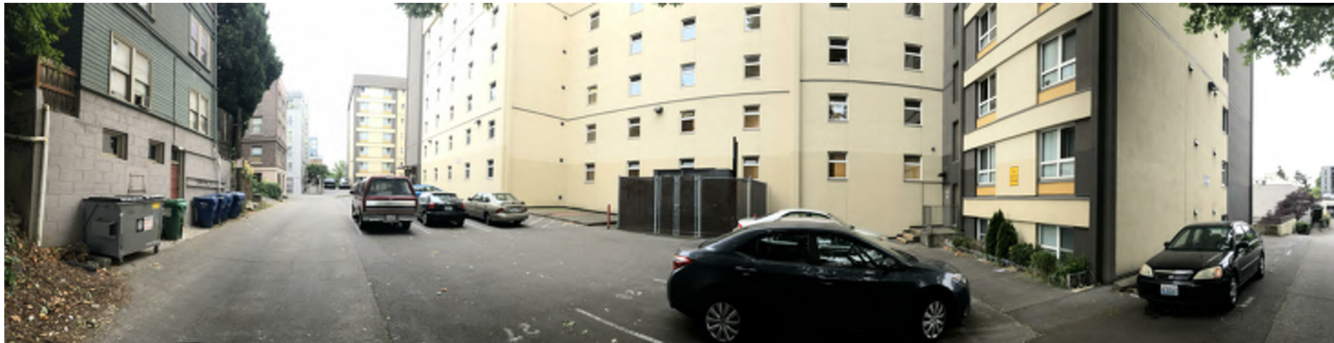
West Structure in Alley Adjacent to Site
