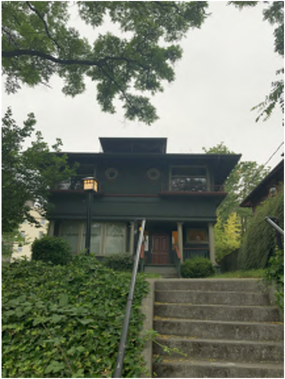
Existing Structure B
