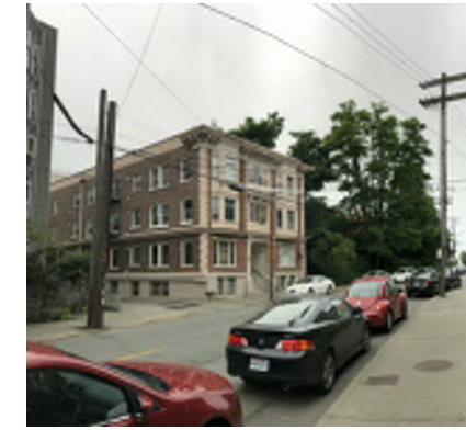
7 - South Adjacent Structure
