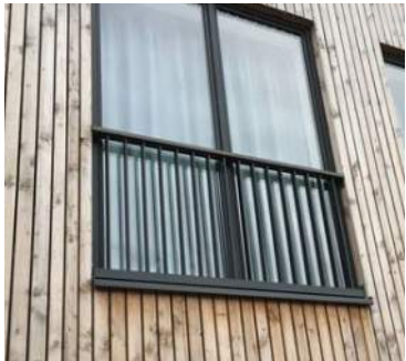
METAL RAILING (G) Painted Black, with Wood-Like Top Rail
