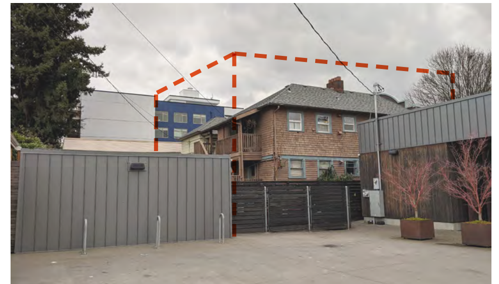
③ VIEW OF SITE FROM N 40TH ST
