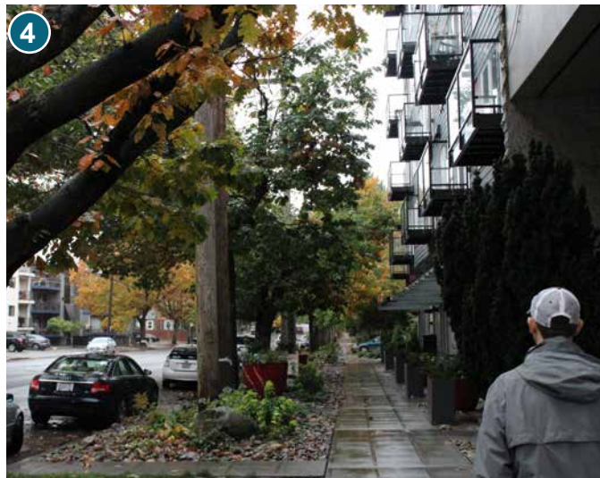
KOI - NW MARKET ST FACADE 6-STORY MIXED-USE RESIDENTIAL
