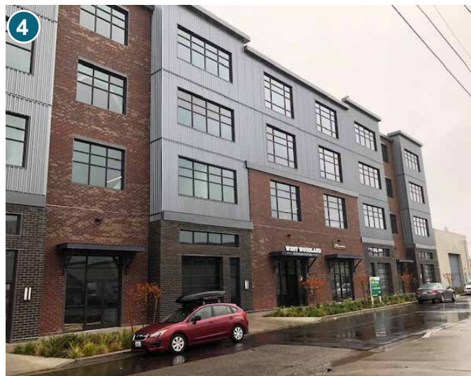
RECENTLY BUILT 4 STORY WORK LOFTS
