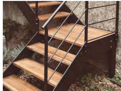
STEEL RAILING (F) + OPEN RISERS
