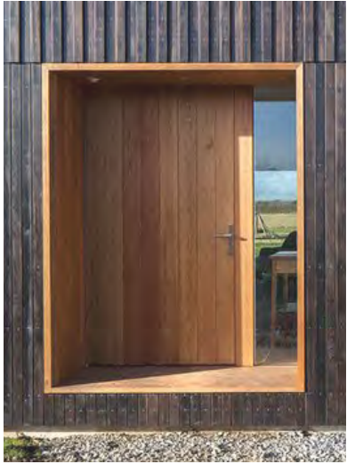
HIGH QUALITY MATERIAL TO HIGHLIGHT ENTRY
