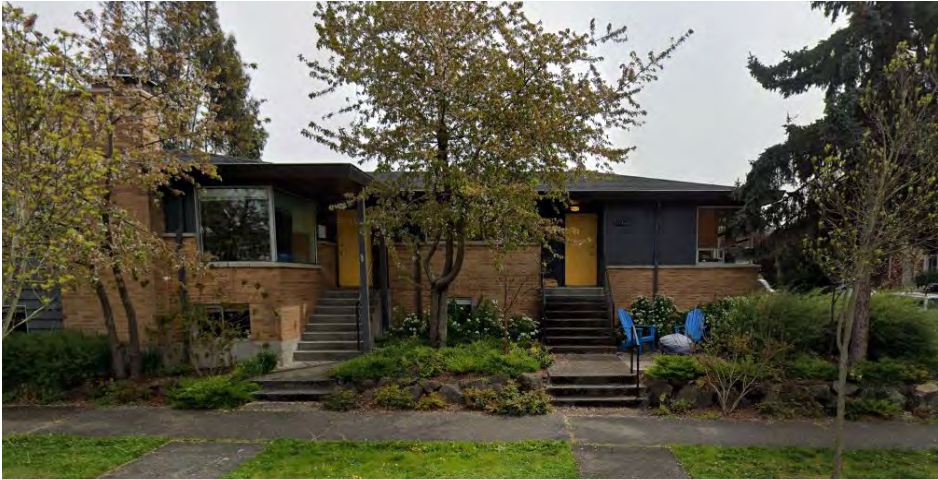
2 STAIRS LEADING TO ENTRY+BRICK AT BASE
