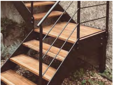
STEEL RAILING (F) + OPEN RISERS
