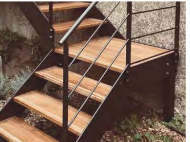
STEEL RAILING (F) + OPEN RISERS
