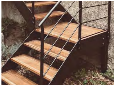
STEEL RAILING (F) + OPEN RISERS
