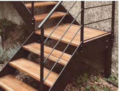
STEEL RAILING (F) + OPEN RISERS
