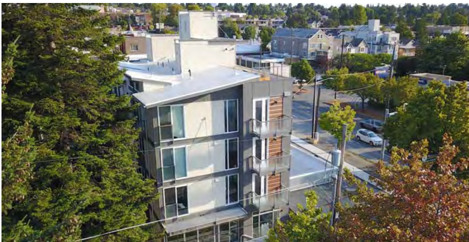
11 SHED ROOF + DECKS
