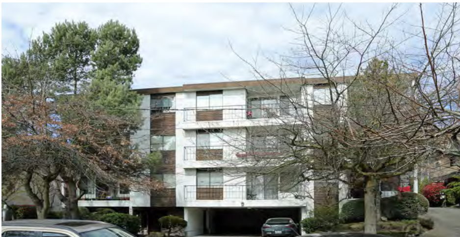
10 STREET FACING DECKS
