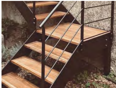
STEEL RAILING (F) + OPEN RISERS
