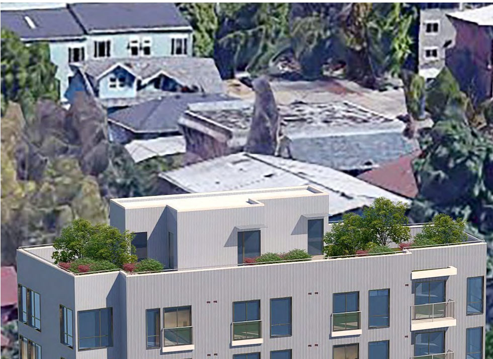
ROOFTOP DECK WITH CONTAINER GARDEN PLANTERS
