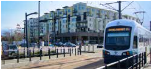
1. OTHELLO LIGHT RAIL STATION.
