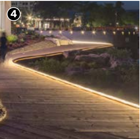
Recessed, continuous linear luminaire to highlight path edge
