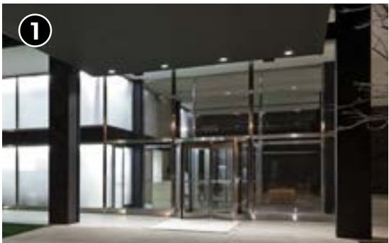
Recessed downlights highlight entries; light source regressed within fixture
