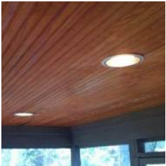
1 RECESSED CAN LIGHTS (SOFFIT)
