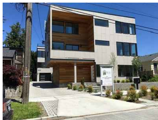
(D) 826 NW 53rd St [(2) single family) & (2) Townhouse] neighboring project site at south
