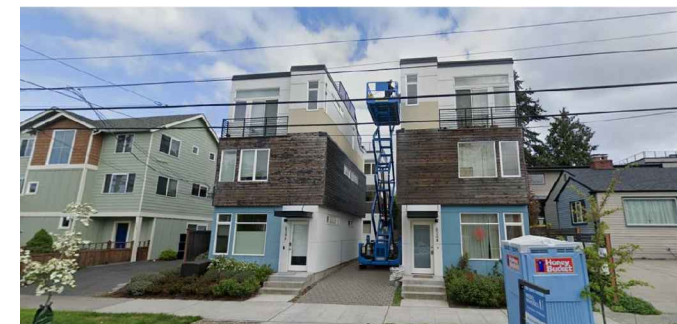
(G) 834 NW 53rd St [(2) single family) & (2) Townhouse] neighboring project site at SW
