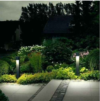
② path lighting along walking paths, parking, and driveway areas
