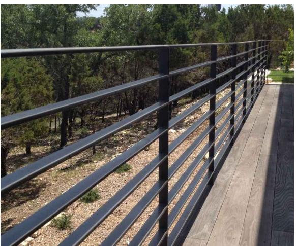
flat bar steel railings ⑤
