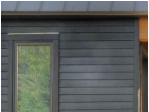
dark framed windows ④
