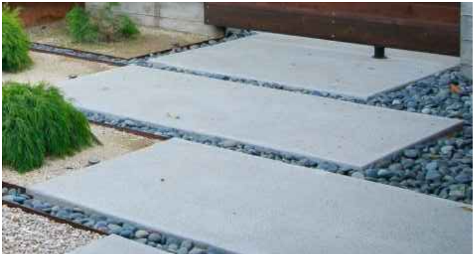
concrete paving w/ gravel strips
