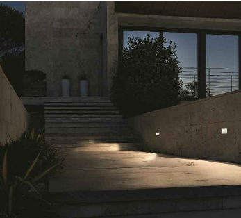
③ step lighting along benches / planters in common areas
