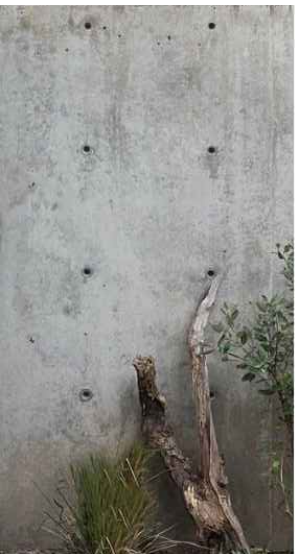
concrete seating, walls, edging
