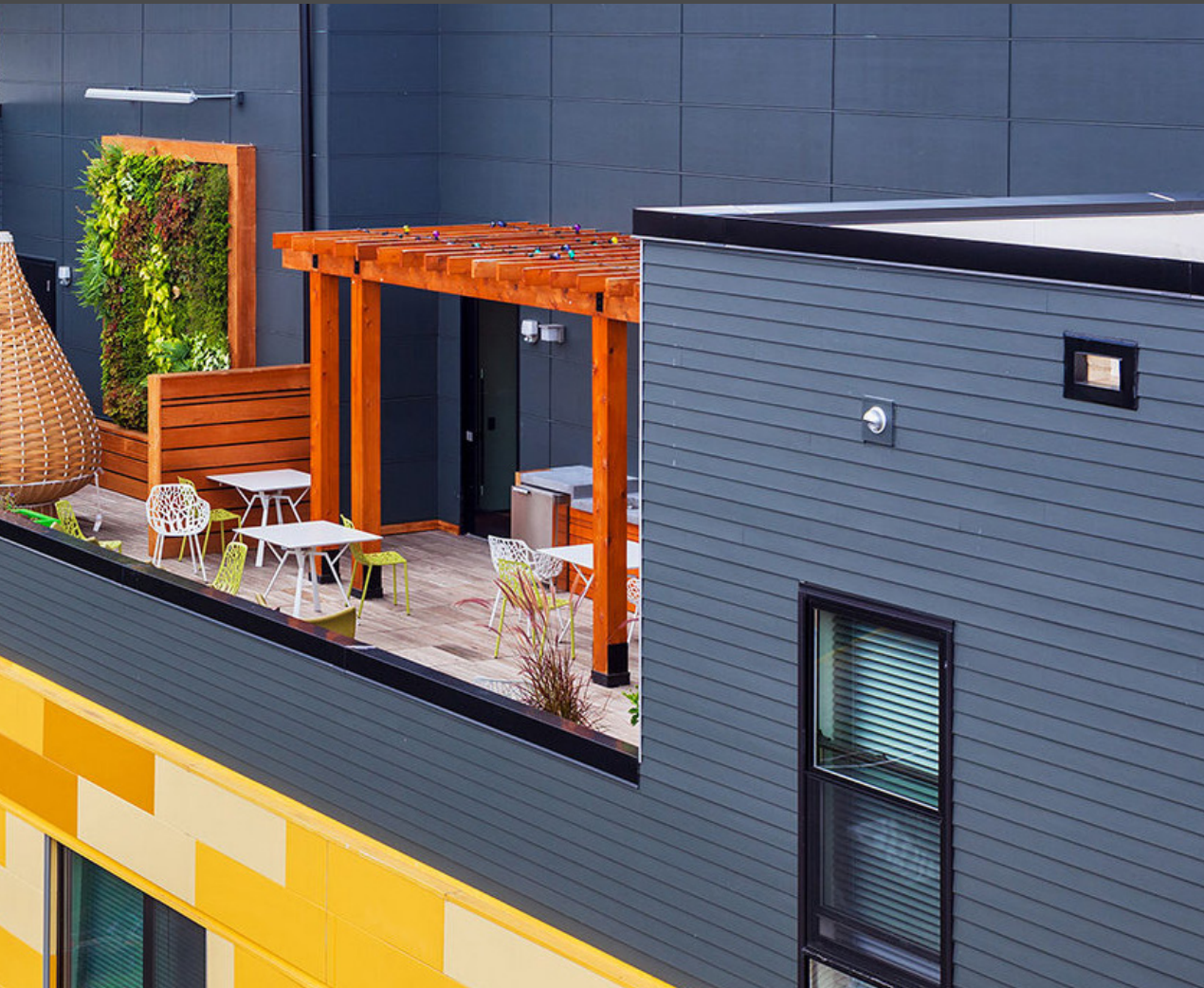
Cementitious Lap Siding facing residential zone
