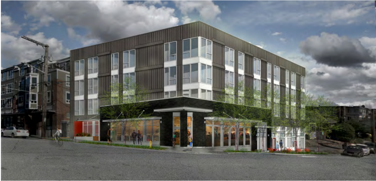
800 5th Ave N (Under Construction)
