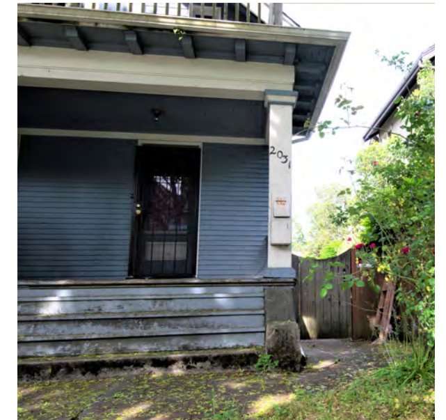
View from Eastlake looking west
