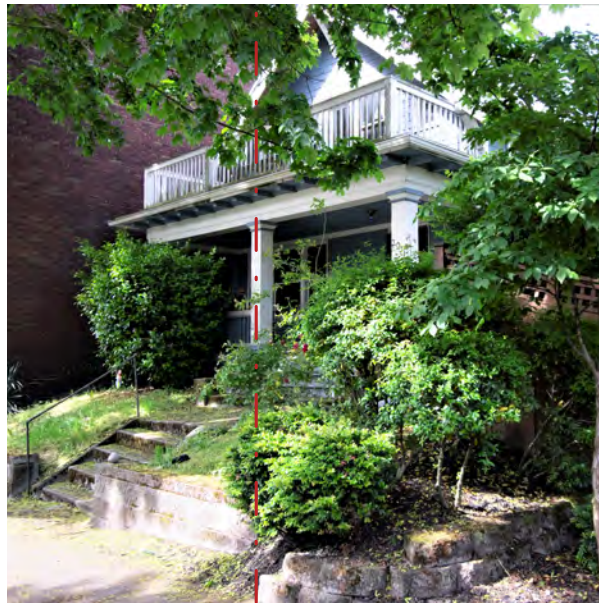
View from Eastlake looking southwest
