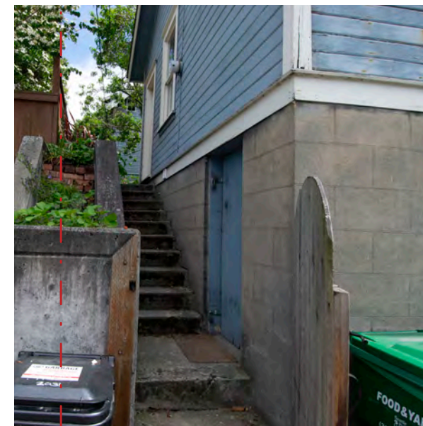
View from alley looking east
