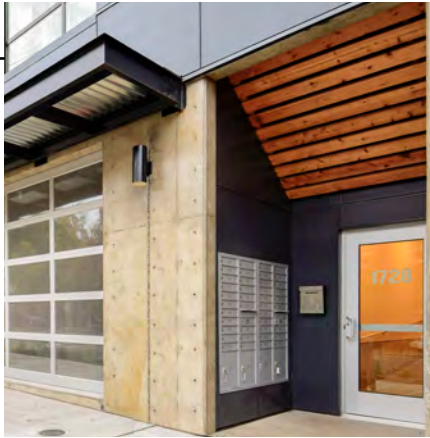
Accent Material at Recessed Entry DC2.D.2: thoughtful application of texture at street level
