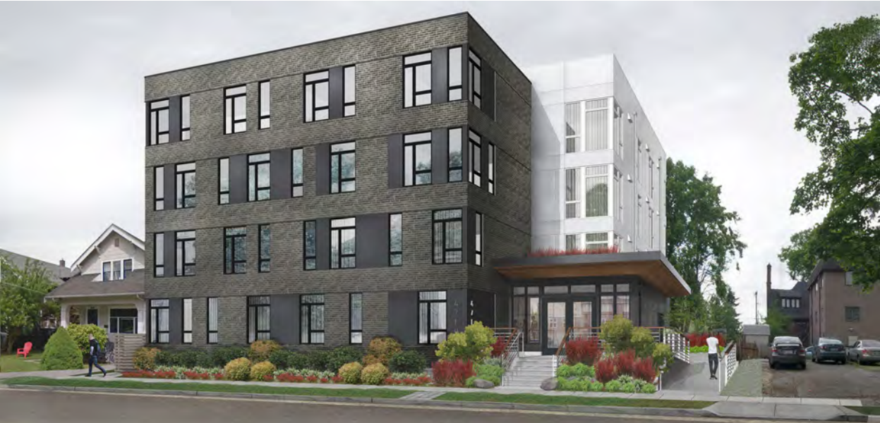
4710 20th Ave NE (Under Construction)
