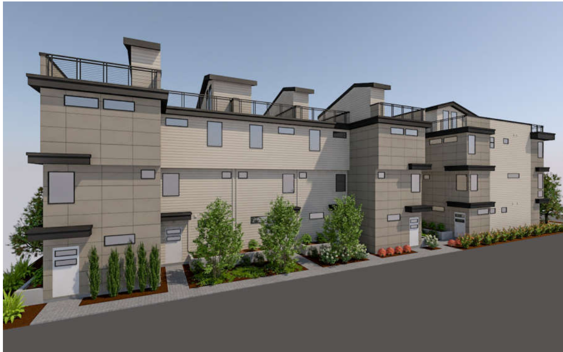
Looking Northeast at Building 2
