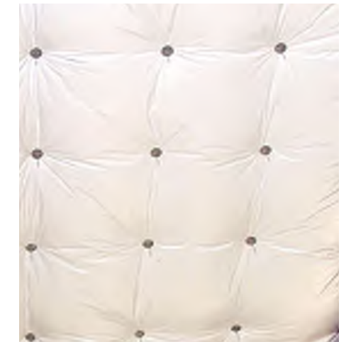
White Facing Stick Pin Insulation (S-06)
