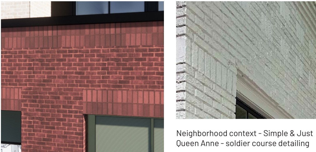
A Proposed Double Soldier course at cornice and lintel Responds to Queen Anne Design Guidelines CS3.II.ii.e+f+i
