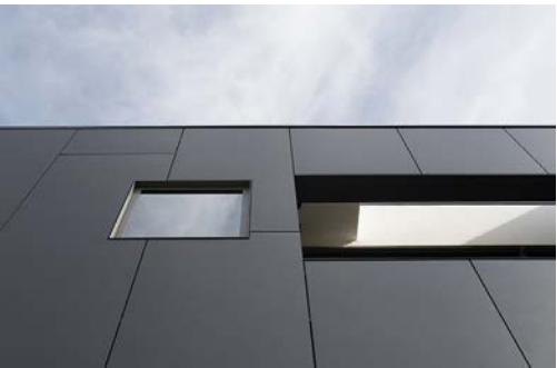
Clean simple detailing, dark metal cladding with dark windows (DC4)
