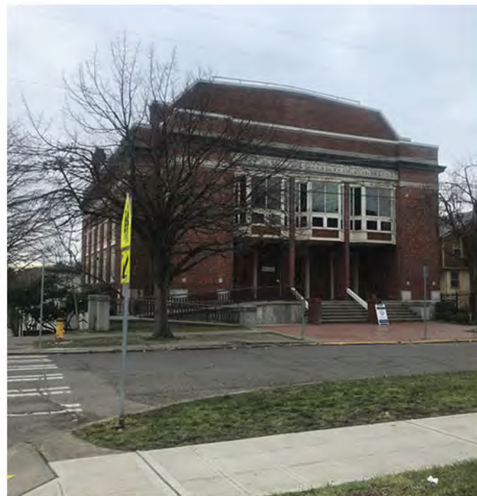
D Present Use: Christian School. Educators and social workers on site. Building built in 1925. Beaux-arts / Neoclassical style. Registered as a National Historic Place. Was once a synagogue.
