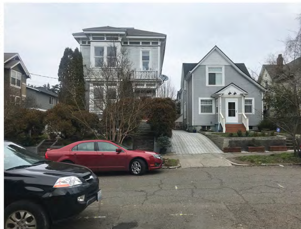
M Examples of early 20th century Victorian architecture at two single family residences. (The one on left is currently a duplex.)
