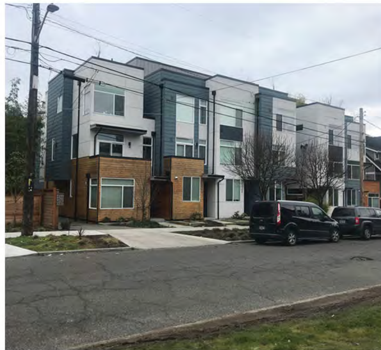
H Example of new townhome construction. Built in 2015.
