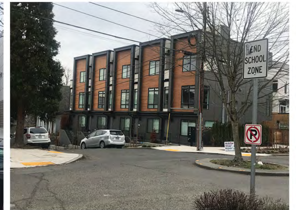
G Example of new rowhouse construction.
