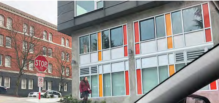
DC4/A.1.1B: Colorful expression through facade features such as these colored panels can be used as accent features or to highlight our wayfinding signage.
