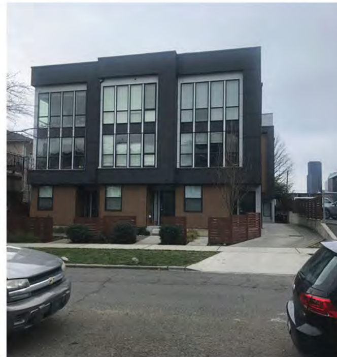
I Example of new townhome construction. Built in 2015. Upper floors have view of Downtown.
