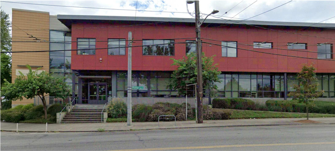
9245 Rainier Ave. S. similar window type, brick, panelized sections
