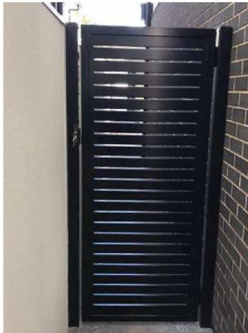
GATE ACCESS TO STAIRS
