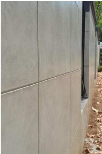
Exposed Concrete reveals
