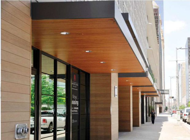
3 RECESSED CEDAR SOFFIT LIGHTING
