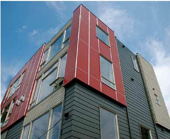
(2) Hardie-Panel Siding w/metal reveals
