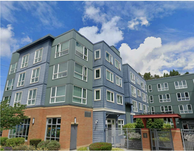
8124 Rainier Ave. S. similar window type, brick, panelized sections
